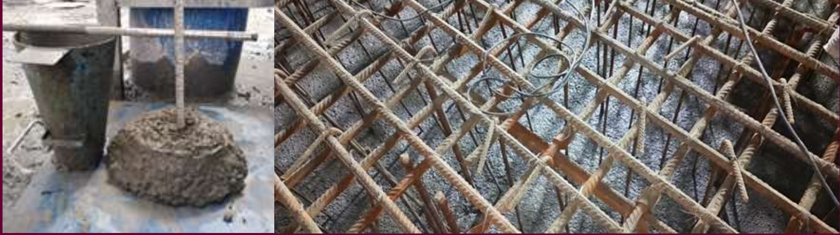
M35 Raft Temperature Controlled Concrete
